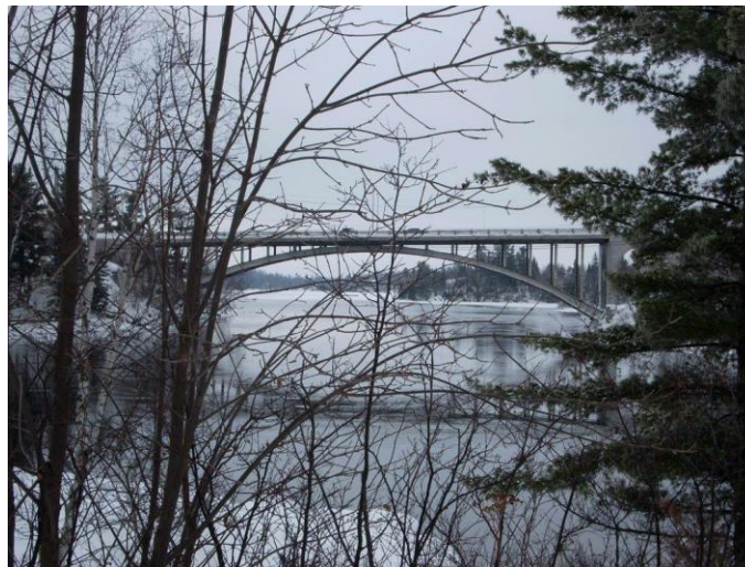
Figure 1: Keewatin Bridge (source: City of Kenora)
